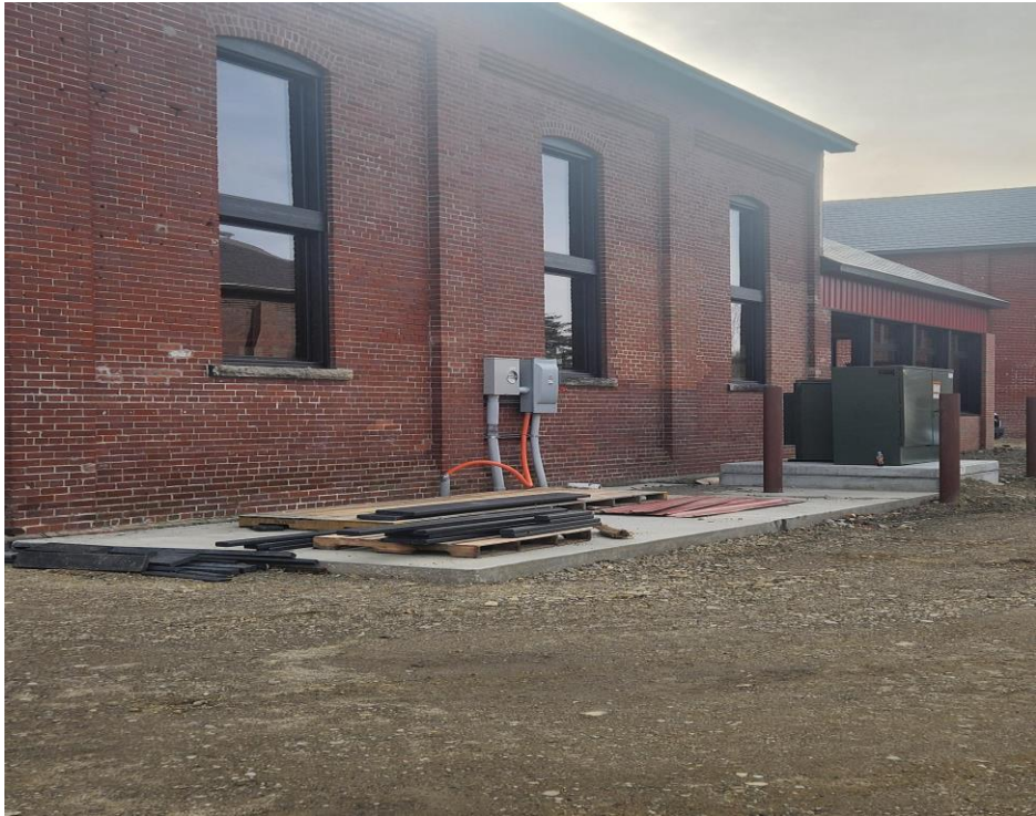
Figure 9. Recommended area for pollinator garden outside the event hall where air conditioning units will be installed.
