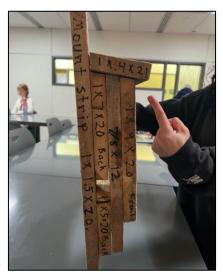
*Figure 22.* Side of bat house. Dimensions (inches) Front: 1x9x20; Roof: 1x4x21 Mount strip: 1x1.5x20 Back: 1x7x20; Back (2): 1x5x20
