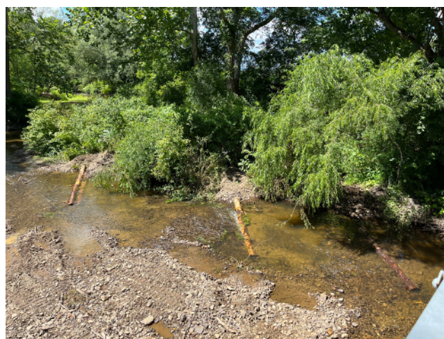
Single log vane deflectors installed at the Woodcock Creek site.
